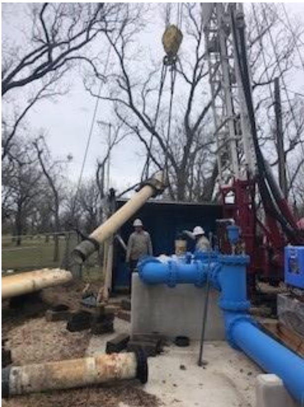
Figure 1: Reinstalling Pump Column
